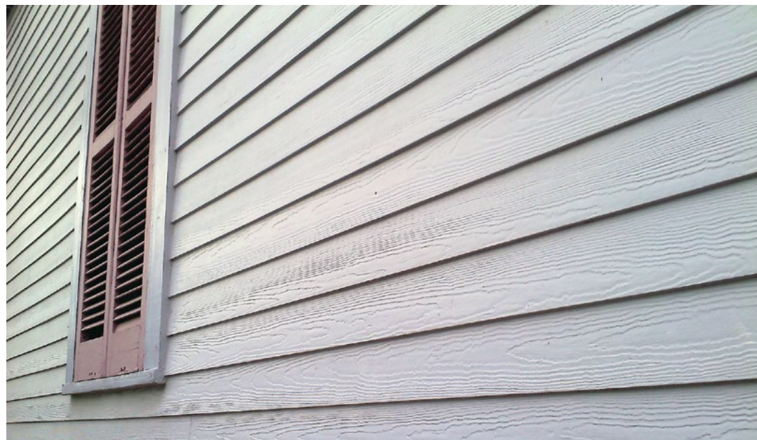
[10] Not Recommended: Cementitious siding with a raised wood-grain texture is not an appropriate material to replace historic wood siding, which has a smooth surface when painted.
